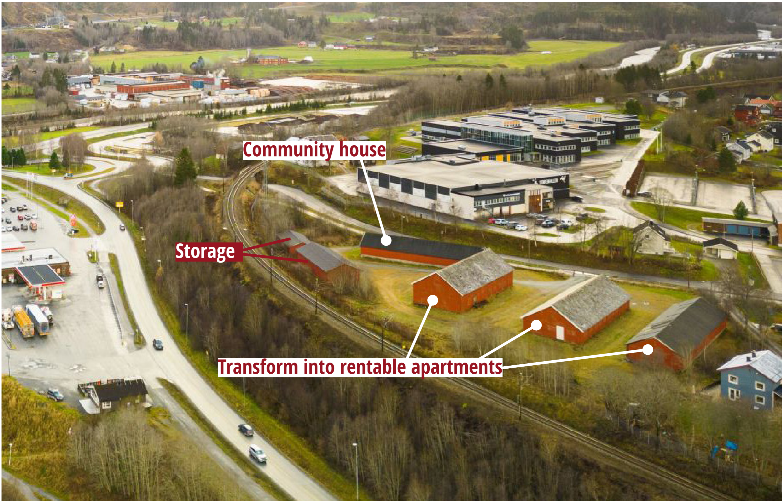
Transformation of the red barracks
